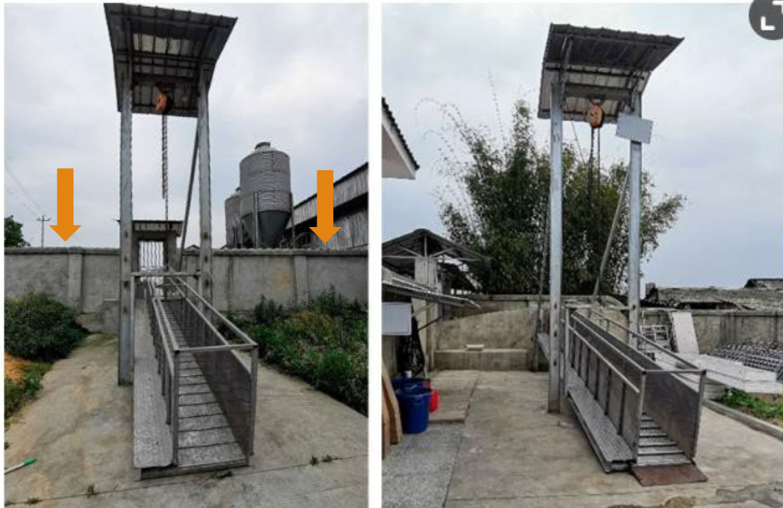
Picture 5. Aluminum open loading chute at the farm perimeter, China. Courtesy of DanAg Group.
