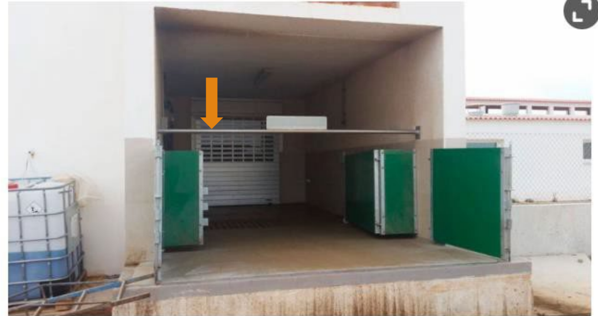
Picture 6. Semi-enclosed loading chute with gates and a horizontal bar to physically separate clean and dirty zones. Courtesy of Agropecuaria Los Girasoles, Spain
